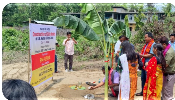
Laying of the foundation stone of a new girls' hostel under PM-USHA
